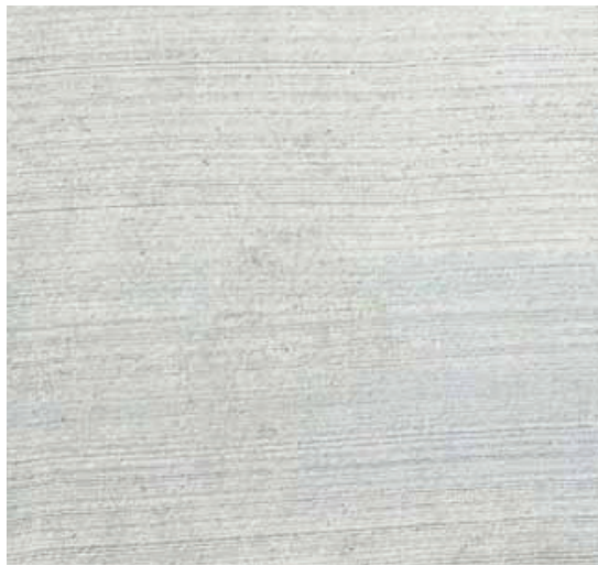
Concrete Paving with broom finish
